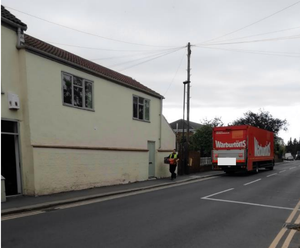
View of the west elevation looking south from Thorpe Lane
