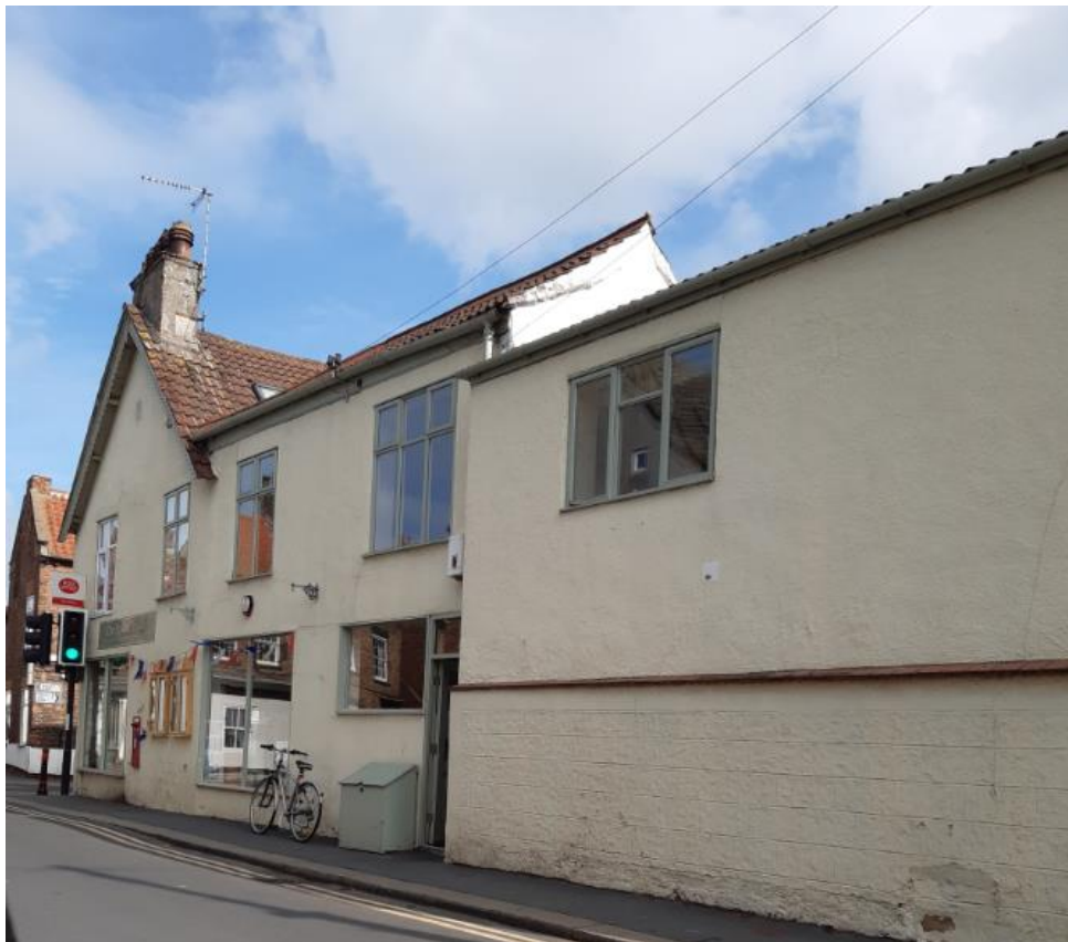
View of the west elevation looking north from Thorpe Lane
